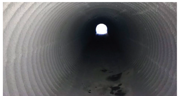
CMP Restored Using The Quadex Lining System
